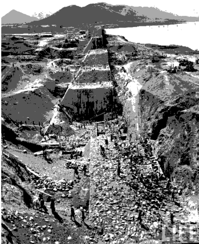
Fig 5.2 : Tungabhadra Dam Construction - 1952
