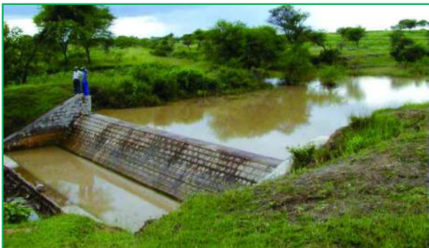
fig-1: Communitybased masonry dam
